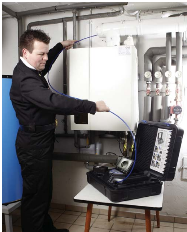
The 360° pan and 180° tiltable color camera head easily negotiates 90° bends.
