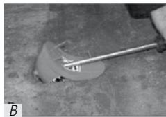
B – Lift void former
