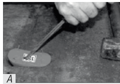
A – Hammer screwdriver (off centre) into void former
