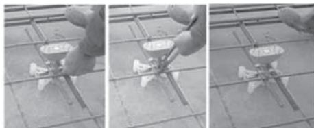
Place two Bars on Barclip of FaceLifter™ Tie-Wire FaceLifter™ in Place FaceLifter™ Secured
